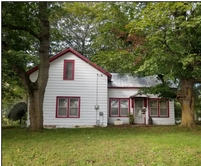
One example of a house in Mecosta.
