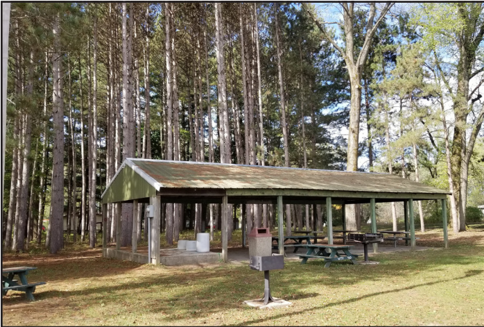
Pavilion at Pine Tree Park.
