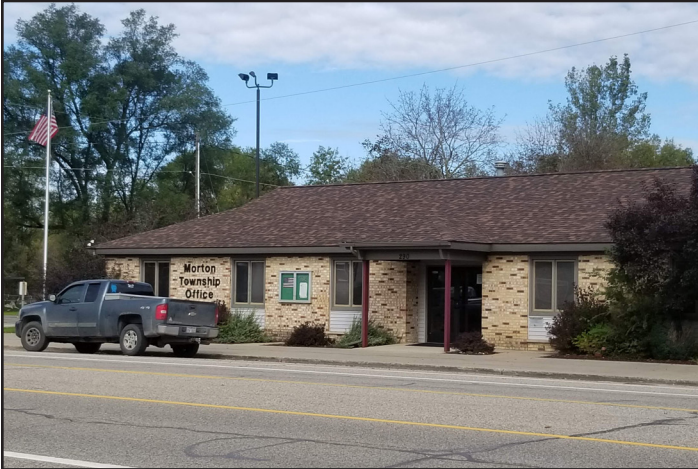
Morton Township Office.
